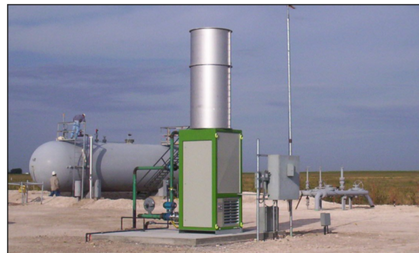
Cimarron's Clean Enclosed Burners (CEB®) are best-in-class in ultra-high Destruction Removal Efficiency (DRE) destroying 99.99% of harmful emissions.
